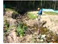
Shell: Natural Reclamation and Erosion Control for Onshore Pipelines, NE British Columbia, Canada
