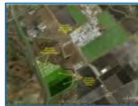
Dow: Constructed Wetland for Waste Water Treatment, Texas, USA
